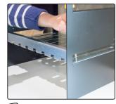
3. Place bottom shelf on side rungs with face toward you pointing upwards. Align holes. Screw shelf to both sides.
