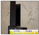
Z. Place bracket INSIDE rack side and screw from OUTSIDE.
