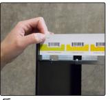
Peel "Rack one, shelf one" rackstrip and line it up with the top shelf cap holes.
